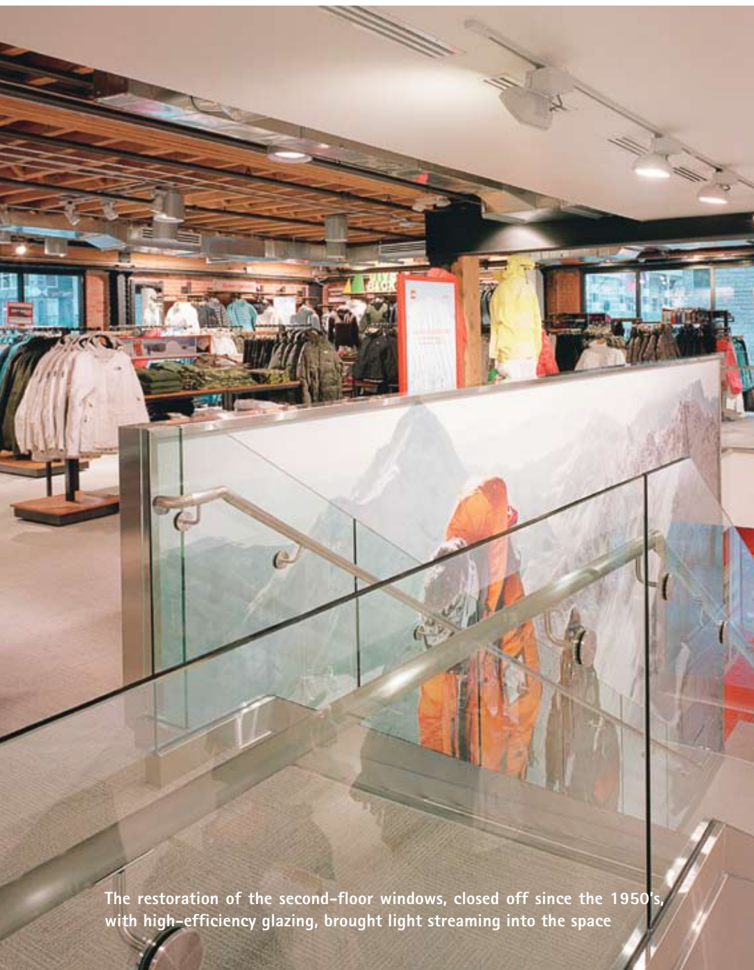
The former department store footprint had to be reconfigured with the large escalators removed in favour of an airy atrium staircase
